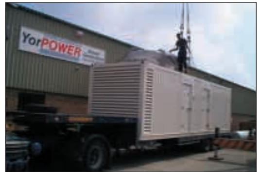
A containerised set being loaded at our site near York
